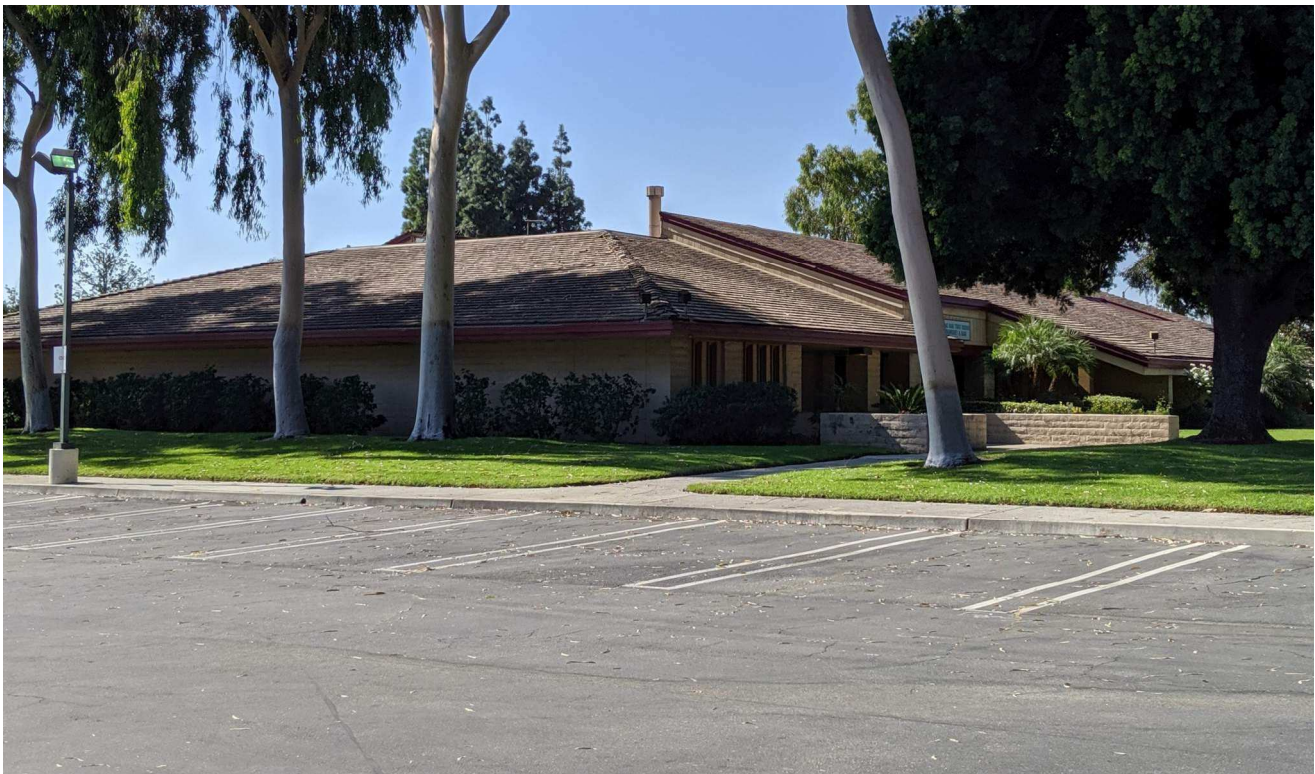
North and East Elevations of Existing Restaurant Building
