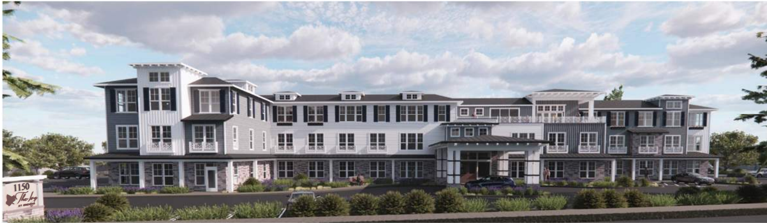
COLORADO BLVD. VIEW
